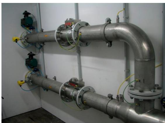
Gas subcontracting of two biogas stations to an entry station with integration of gas analysis and accounting of the gas based on thermal input.
